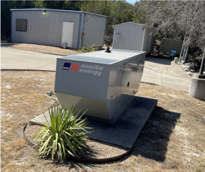
Figure 6 – Propane Generator
