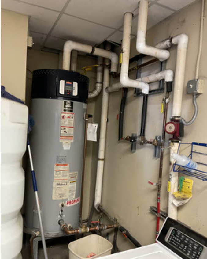
Figure 14 – Water Heater
