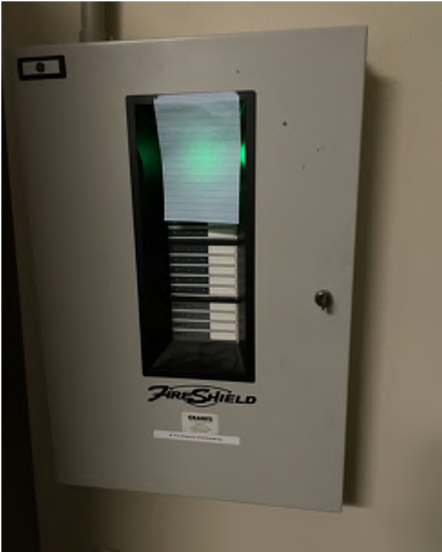
Figure 17 – Fire Alarm Control Panel
