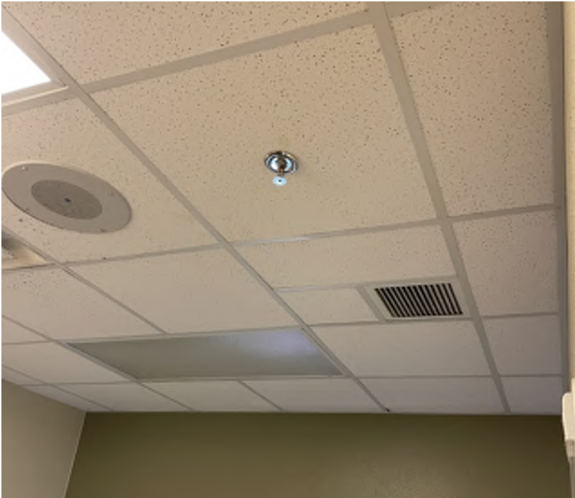
Figure 11 – Dorm Room Ceiling
