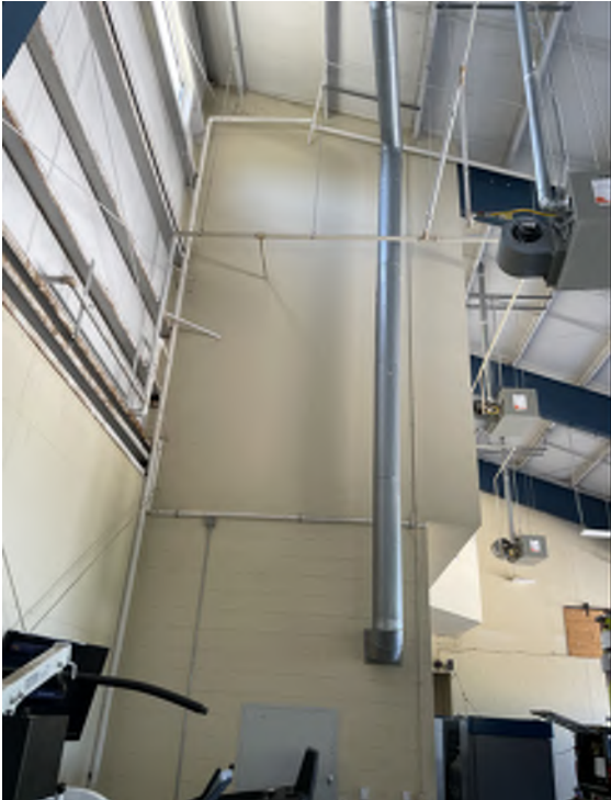
Figure 13 – Back of mezzanine (Dumbwaiter will require removal)
