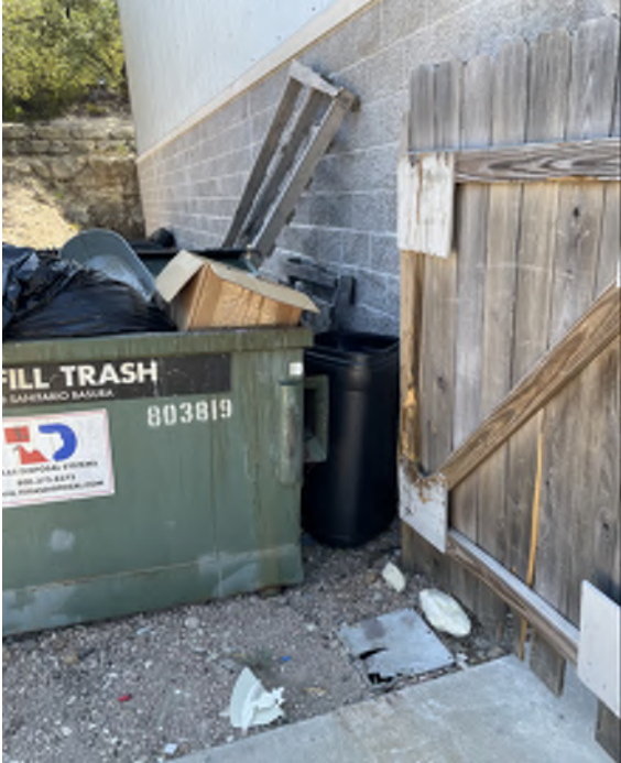
Figure 16 – Side of building with unknown ground enclosure (ID required)
